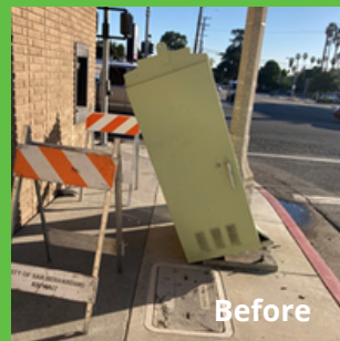
Traffic signal controller cabinet damaged due to traffic collision at Highland Ave & Arrowhead Ave
